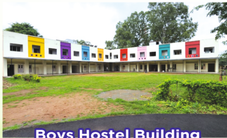
Boys Hostel Building
